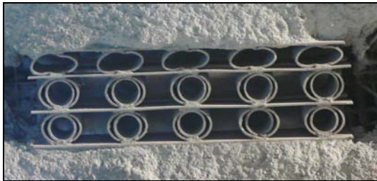
Picture 12: Honeycomb set between 2 lattice girders
