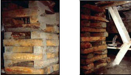
Picture 1: timber cribs
