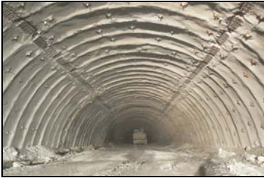
Picture 6: Support with stress controller, System Honeycomb
