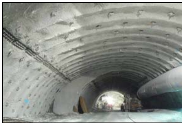
Picture 17: First use of Honeycomb in Tauerntunnel
